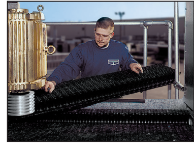
Water Saver Drift Eliminator
