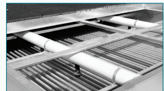
Drift Eliminators Removed for Coil Inspection
