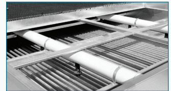
Drift Eliminators Removed for Coil Inspection
